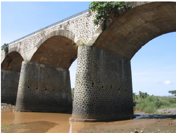
One of the oldest masonry arch bridge :- Birr wuha bridge
