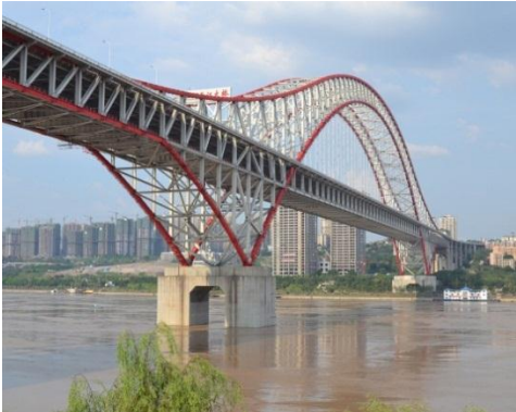
552 mt long steel arch bridge, 2009, China
