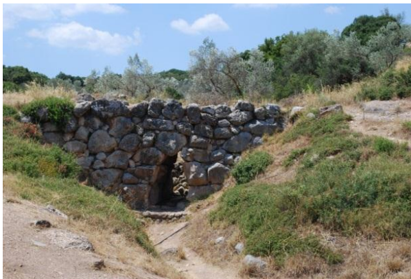
The Arkadiko Bridge, 1mt clear opening and 22 mt total length,
