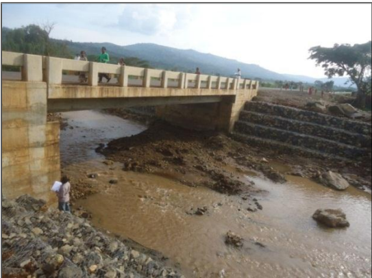
Example of bridge pictures before and after replacement.
