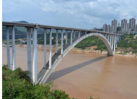
420 mt long Concrete arch bridge, 1997, China
