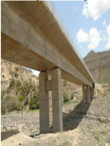
Wakela River Bridge
