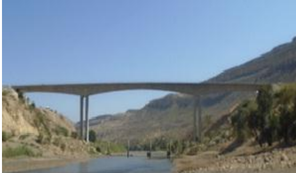
Abay No. 8 Bridge
