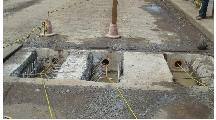
Anchor blocks reinforcement grouting
