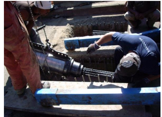
Cable tensioning
