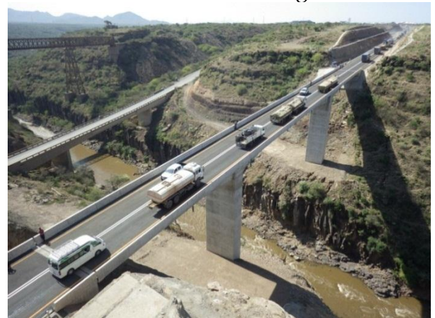
New Awash bridge
