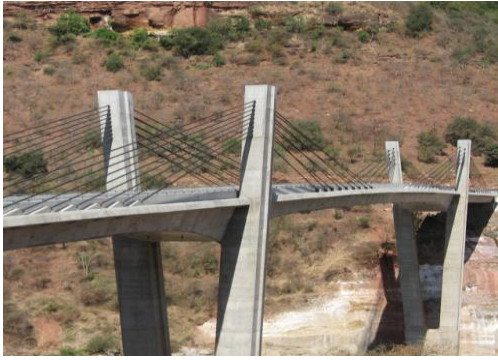
Abay No. 6 Bridge
