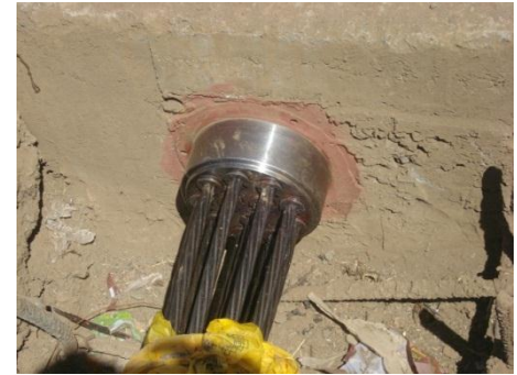
cable tensioning
