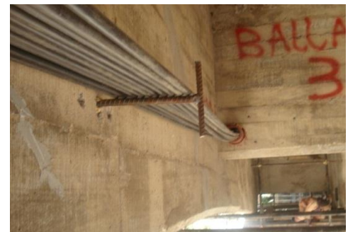
Externally tensioning cables
