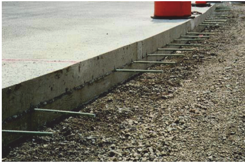
Figure 2-1: Tie bars in place to connect to parallel concrete slab
