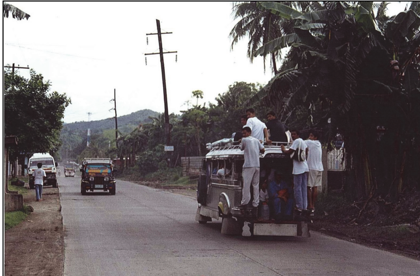
Figure 1-2: Jointed unreinforced concrete road in a semi-rural area with a shoulder of unbound material: Design Standard DC6, Traffic Class T6
