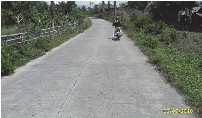
Figure 1-3: Low volume jointed unreinforced concrete road in a rural area- Design Standard DC5, Traffic Class T2
